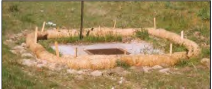
Figure 182. Inlet protection wattle (ITD 2014).
