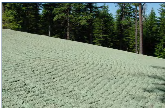
Figure 137. Exposed soil temporarily stabilized by roughening the surface ( North Idaho Hydroseeding ).
