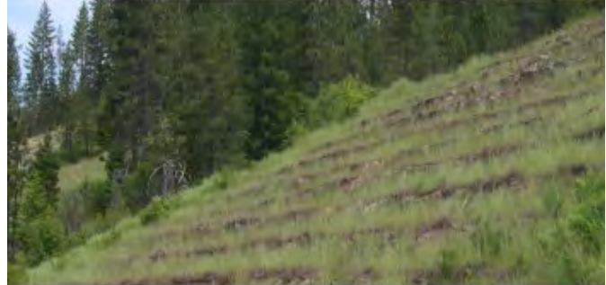
Figure 140. Terraces incorporated into the grading plan (ITD 2014).
