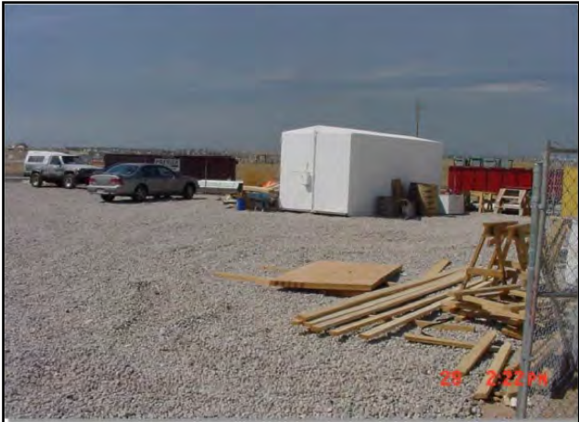
Figure 98. Construction staging area (Colorado UDFCD 2010).
