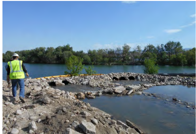
Figure 143. A rock check dam reduces runoff velocity.
