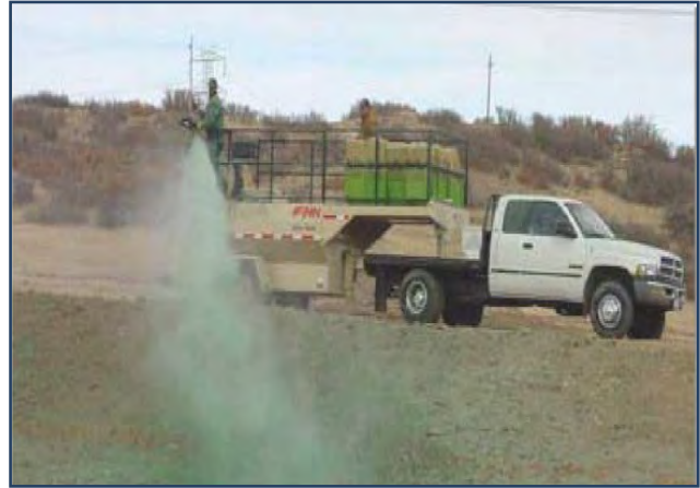
Figure 128. Soil stabilizer application in Douglas County, Colorado (Colorado UDFCD 2010).
