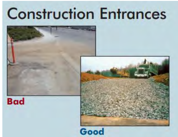
Figure 102. Stabilized gravel construction entrance examples (EPA 2003).
