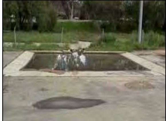
Figure 117. Vehicle and equipment wash area (CALTRANS 2003).
