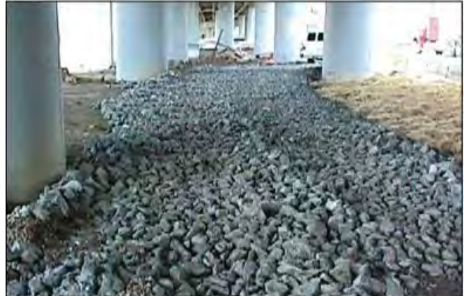
Figure 108. Temporary construction access road (ITD 2014).
