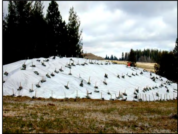
Figure 114. Covered stockpile (ITD 2014).
