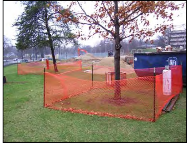
Figure 99. Preserve vegetation (Elkhart County SWCD 2007).
