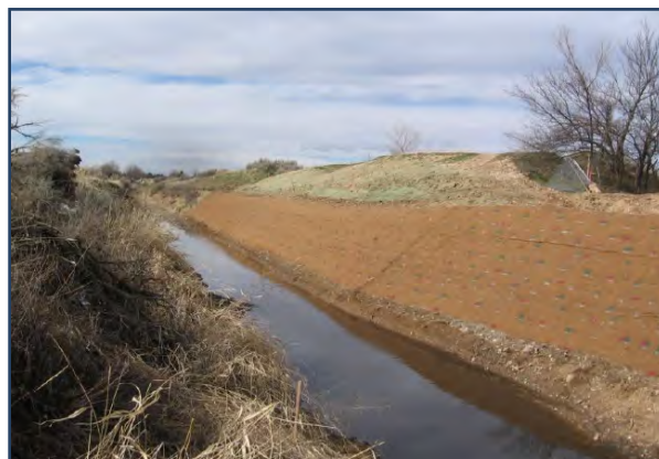
Figure 123. Geotextile channel lining (ITD 2014).
