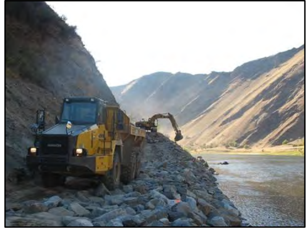
Figure 129. Riprap stabilization of the Salmon River Road, Riggins, Idaho.
