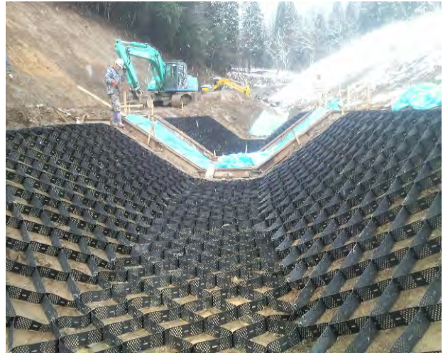
Figure 146. Geocells can be filled with soil and vegetation, rock, or concrete.
