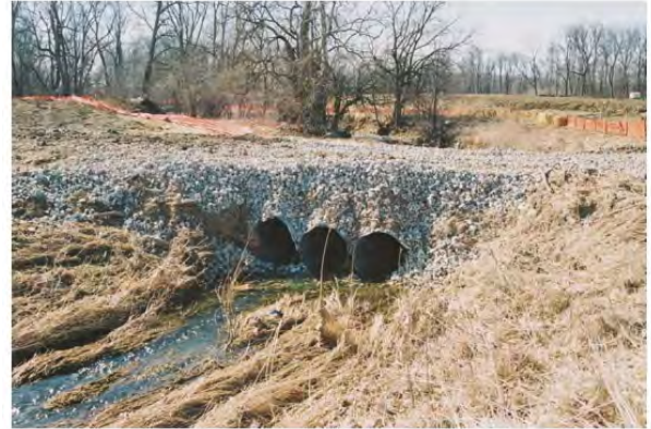
Figure 149. Temporary stream crossing using culverts (Ohio EPA 2014).
