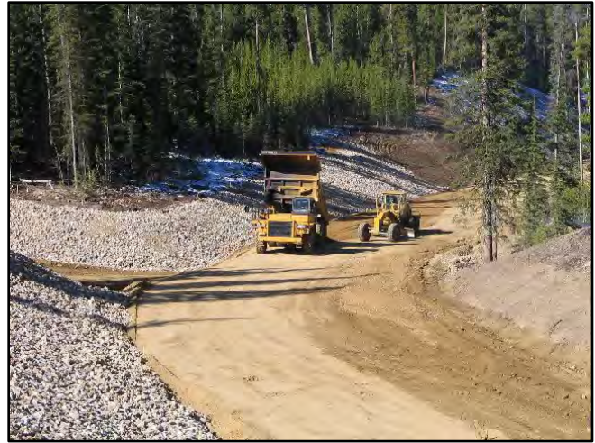
Figure 83. Placing new topsoil on Pioneer Mountain scenic byway, Orofino, Idaho ( Debco Construction ).
