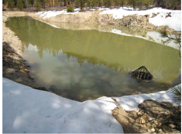
Figure 160. Sediment basin designed to remain at a certain depth.
