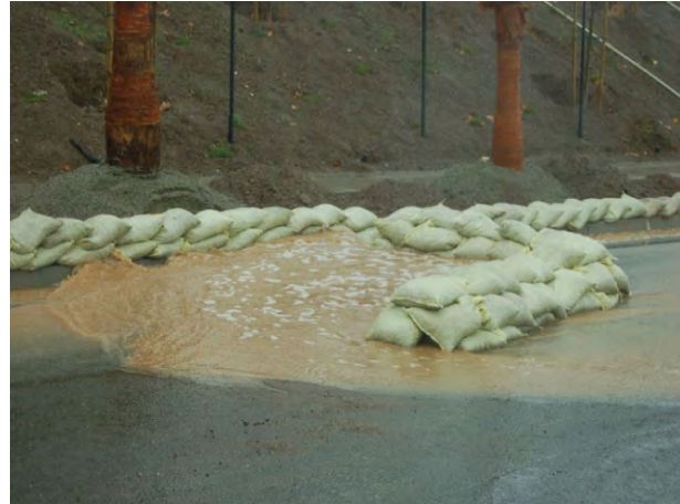
Figure 171. Gravel bag berm ( Natural Building Blog ).
