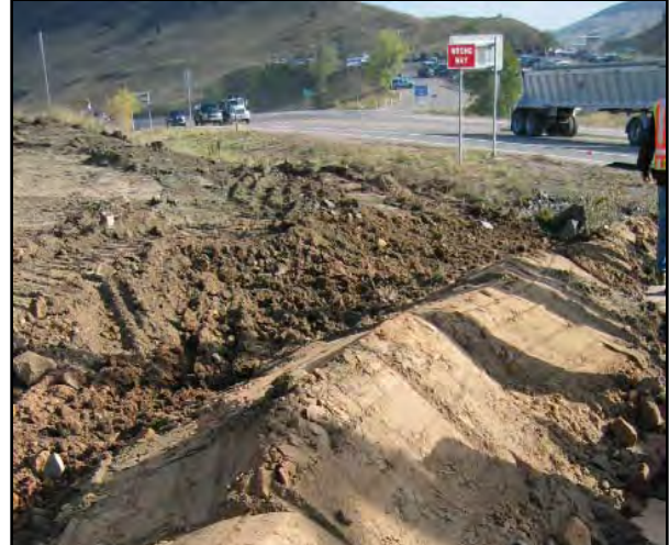
Figure 168. Earth dike diverting flows at a construction site (CALTRANS 2003).
